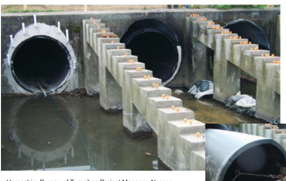
The New Hampshire Bureau of Turnpikes Project Manager, Nasser Yari was concerned about the condition of an existing multi barrel corrugated metal culvert system that was installed in the 1960's. These culverts located on I 95 under Portsmouth Circle in Portsmouth, NH carry water to the Atlantic Ocean and are under very deep fill. Portsmouth Circle is also a major traffic circle controlling the access for Route 1 Bypass North & South, US 4/NH16/Spaulding Turnpike and IO5
